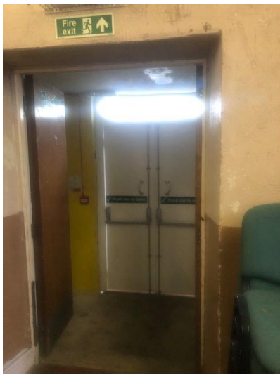
New front door / fire exit
